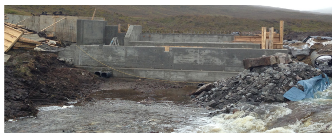
Chore a Bhalachain Intake construction
