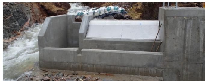
Allt Dubh Intake and Bypass under construction
